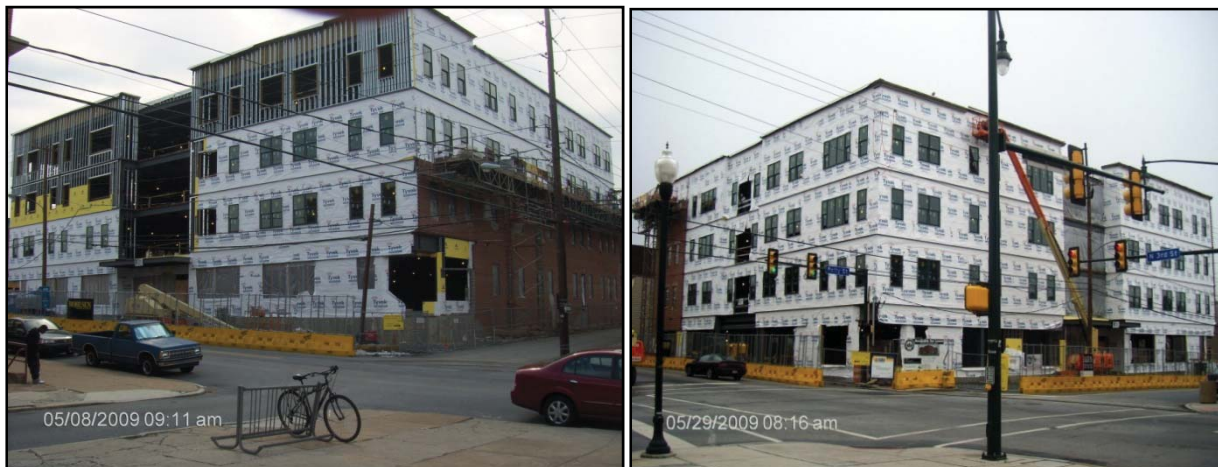
Figure 11-Exterior Façade Construction
