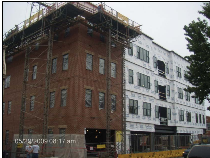
Figure 10 –Installation of the Exterior Wall System
